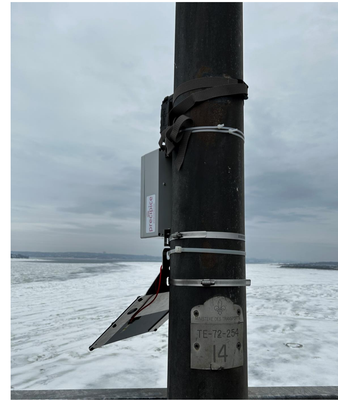
Figure 2: GNSS-IR sensor on the Île d'Orléans bridge in Québec, Canada.
